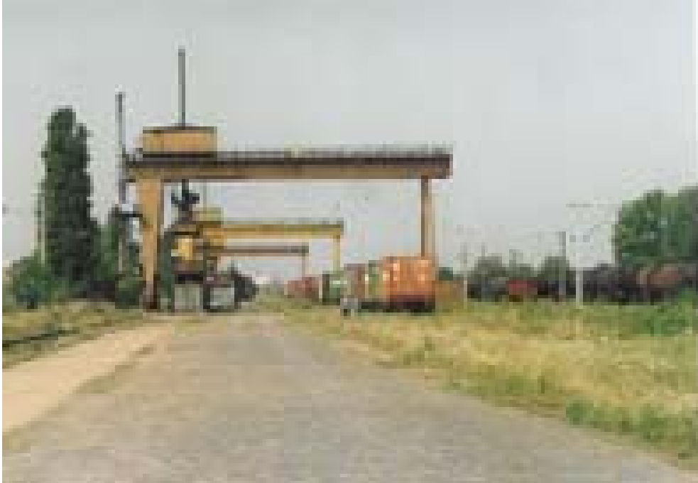
Figure 1-8 Typical terminal layout in Romania
